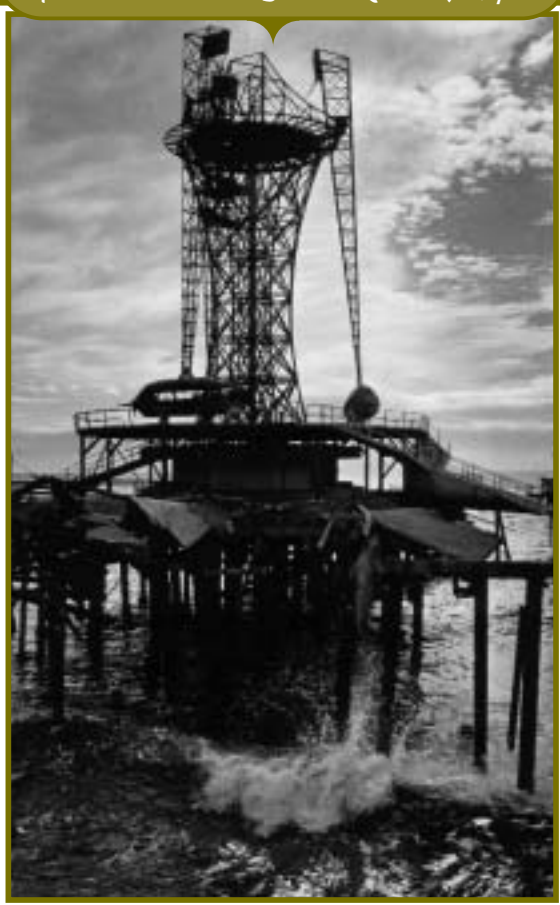
the ocean park pier in the process of being demolished, 1974
